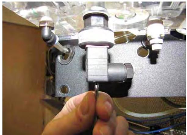
Fig. 36 Loosening fixing screws on the sensor plug
