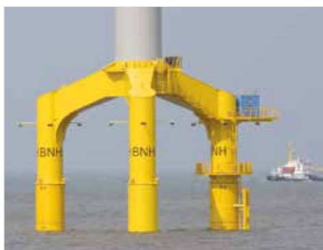
▲ Offshore wind turbines levelling: Enerpac's synchronous lifting system was the solution for leveling support cross pieces on 80 wind turbines.
