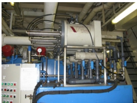
Biological waste water treatment on board of pipe lay vessel "Lorelay" (HMSA)
