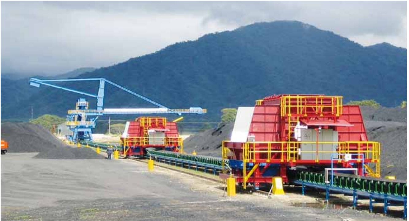
mineral deposits conveyor
