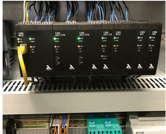
CMS modules installed in the control cabinet.
