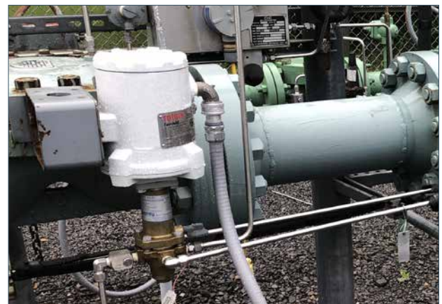
PAX 1 installed in pressure control and metering stations for natural gas distribution
