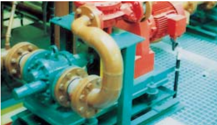
Gear pump T-GKGM in printing-ink installation
